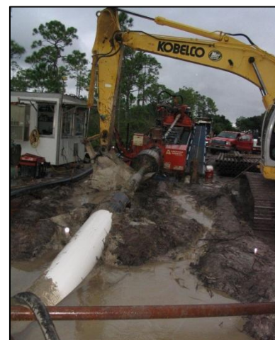
Emergence of FPVC® from HDD pit
